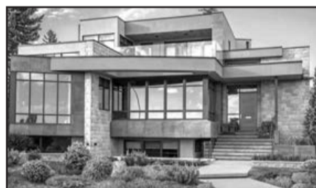
Fire resistant home construction is now at the forefront of discussion for architects and builders alike.
